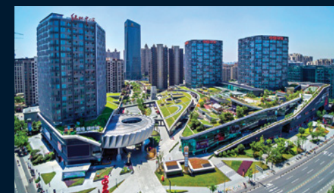
Shanghai Greenland Centre, China
